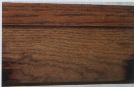
Photo.7: The SOY-Gel cleaned the surface of the oak moulding ready for re-finishing
